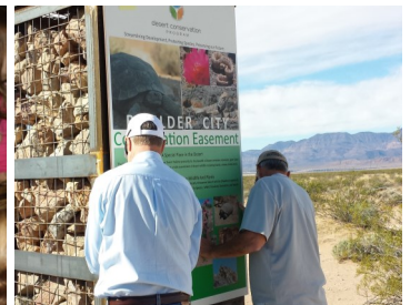
Installation of kiosk at the Boulder City Conservation Easement
